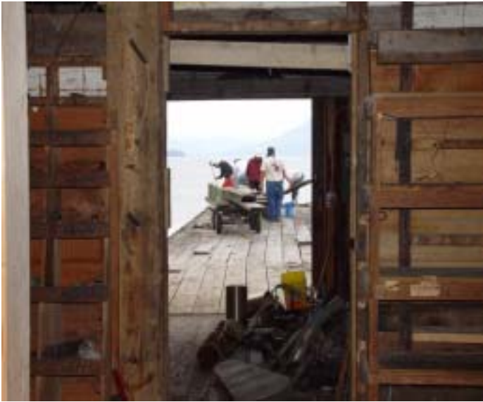
Above: Hoonah workers renovating the Pt. Sophia cannery building and dock
